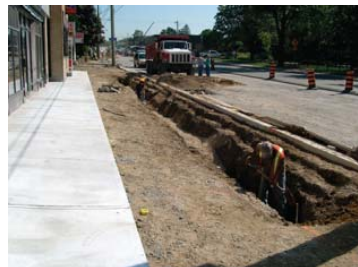
Continuous soil trench under construction
