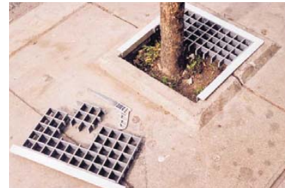
Optional protective tree grate being installed
