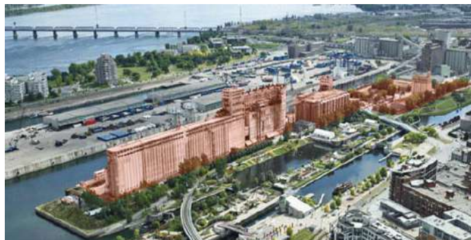
Figure 78: Redevelopment in Quartier De L'innovation
