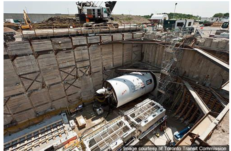
2013 Holey Boring Machine at Sheppard West Station driving north Courtesy of Railway Technology and Toronto Transit Commission https://www.railway-technology.com/projects/toronto-york/?cf-view
