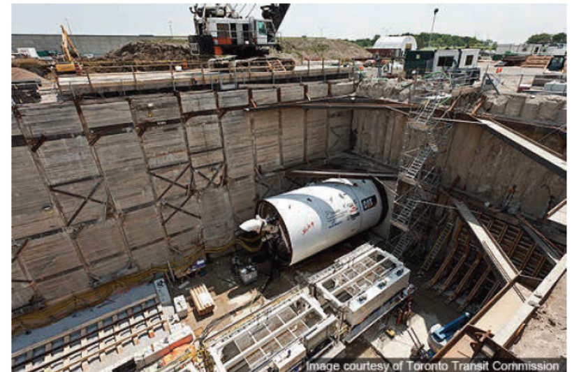
2013 Holey Boring Machine at Sheppard West Station driving north Courtesy of Railway Technology and Toronto Transit Commission https://www.railway-technology.com/projects/toronto-york/?cf-view
